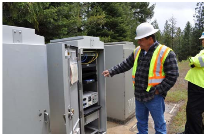
Figure 11: ASWC in Spring Garden ITS Cabinet, as shown by Ian Turnbull
